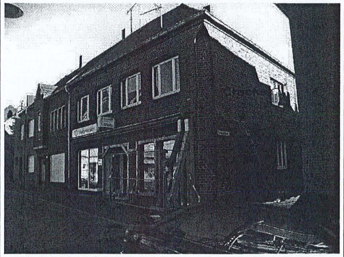
Figure 8. Building that had to be torn down because of the damages caused by ground heave
